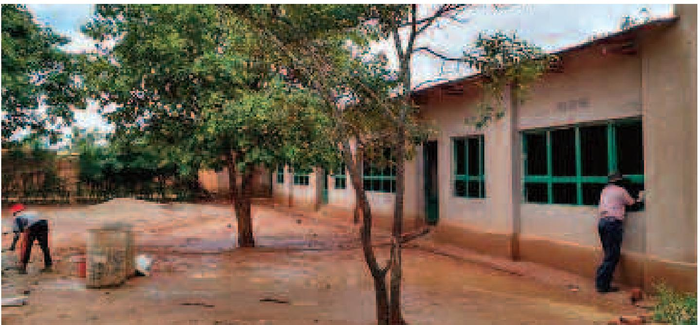
The final stage of construction is captured for the three large new classrooms. Puma (at right) is installing glass in the windows. The classrooms form part of the 500+ meter wall around the campus.
