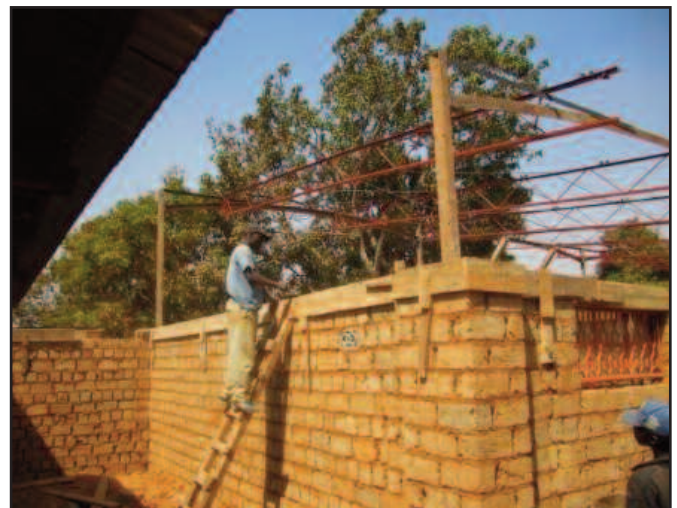
Walls are built but the workshop needs a roof to protect the adobe bricks.
